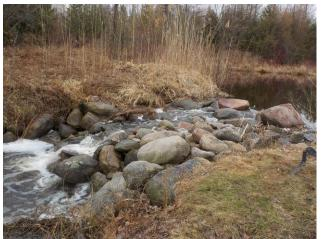
Migratory barrier to fish passage. This is also the water outlet control for the pond.
